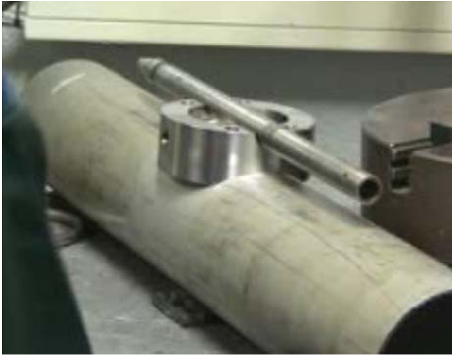
Figure 3-4 Installation of Pasve pH body C in horizontal pipe
